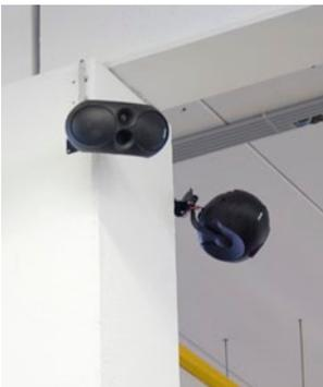
This loudspeaker series comes with an optional special angle bracket.
